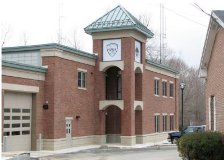
The entrance to the new fire station in Shrewsbury Center. See our website ( http://www.shrewsburyalumni.org ) for photos that Bill Yeomans of the town Historical Society took as the old fire headquarters on the site was razed.
